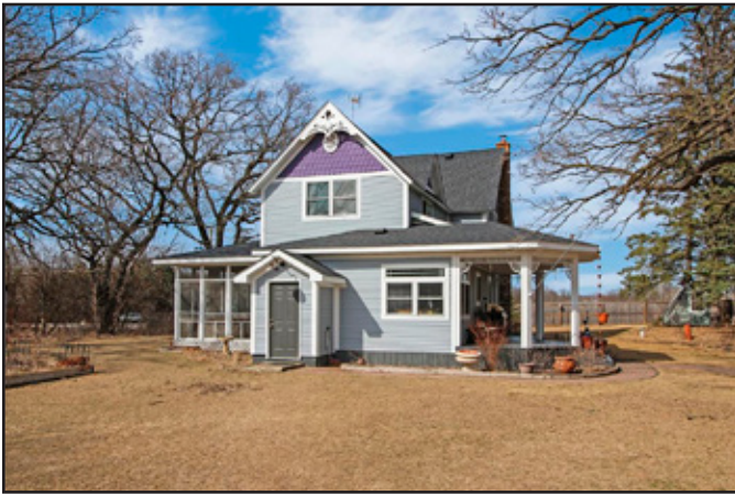
Separate exterior entrance direct to the lower level
