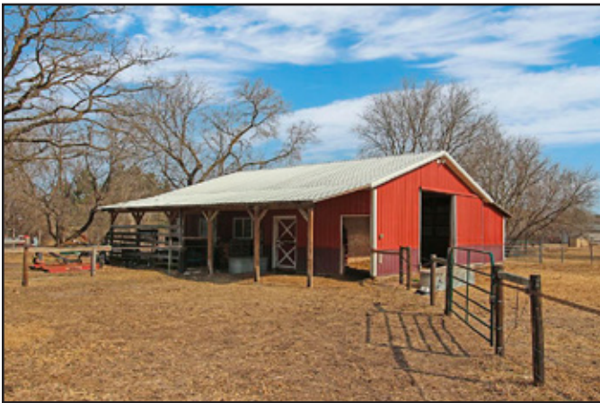
40'x30' horse barn with a lean-to on both sides
