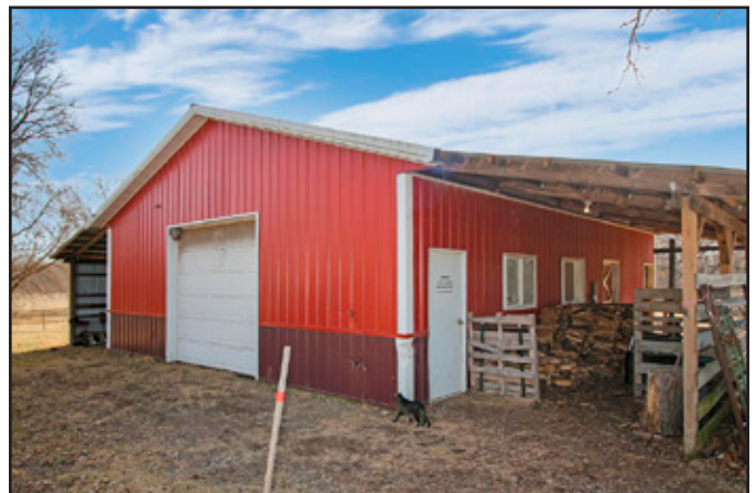
40' x 10' lean-to on both sides of the horse barn
